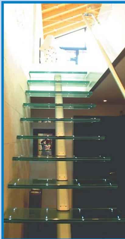
**Fig. 2 - Transparent powered LED stair containing LED film from SUN-TEC. EVA type lamination by Sofraver, Switzerland. Powered @ 24 VDC, 20 mA per glass**
